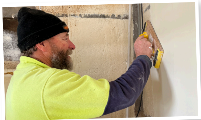
Carpenter Tony Woods refurbishing one of the units.
