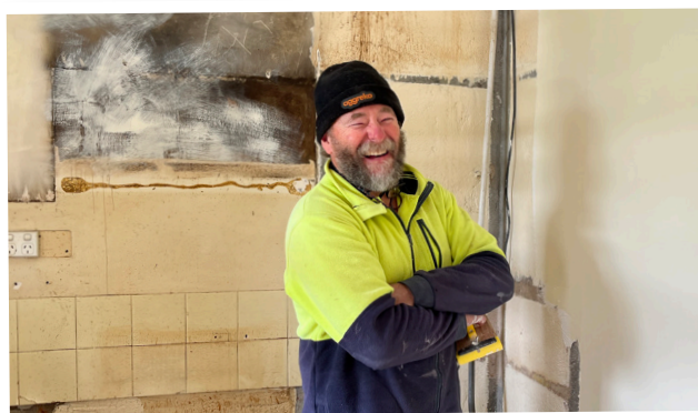
Carpenter Tony Woods has been one of the local contractors doing an amazing job refreshing the units ready to welcome new residents.
